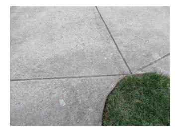
• Heaving/Settlement. Sections of the concrete flatwork have heaved or settled relative to their adjacent sections, creating trip hazards. Americans with Disabilities Act (ADA) defines a trip hazard as any vertical change of ¼" or more at a joint or crack in a walkway surface.
